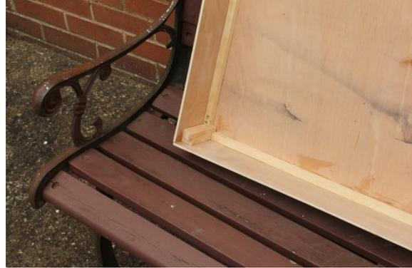
The corners are supported by a pine corner brace, again screwed and glued.
