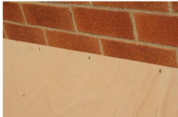
The pine is glued to the board and additional supporting screws fixed through the top of the board.
